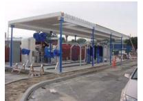
**Paint Booth:** The Fleet Services Division took over the paint booth at the City Service Center to re-paint vehicles. The Division brought the paint booth up to compliance by changing all required filters, lighting, and obtaining all of the required permits to operate.
