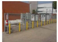
The station consists of two fast-fill pumps, and ten slow-fill pumps. There are two compressor units, and a de-fueling station. The City currently has 12 vehicles that are dedicated CNG.
